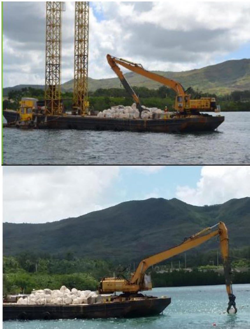
Figure 17. Limestone boulders from a quarry on Guam were transported to a coral translocation site by barge and placed underwater at the selected site (Source: NAVFAC 2018).
